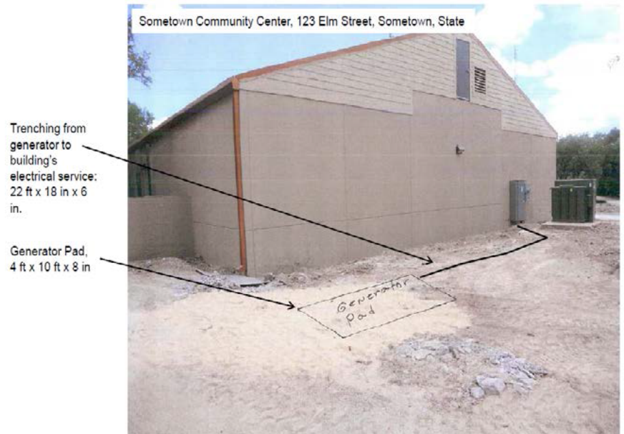
Figure 4. Ground-level photograph showing proposed ground disturbance area.
